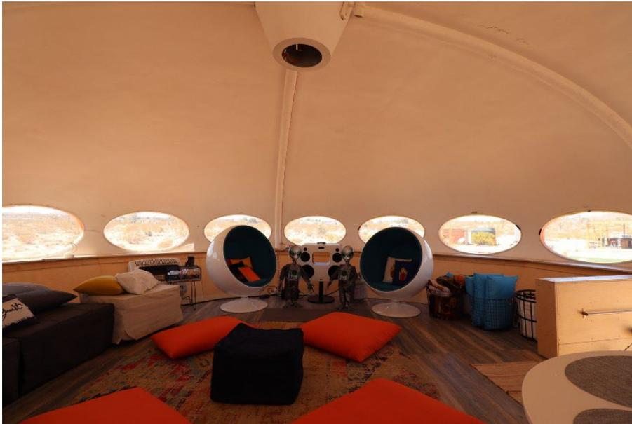
**Photo 10** Replacement birch wainscot and laminate flooring, view northwest and down
